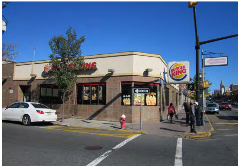
Sidewalks along Bergenline Avenue Are Narrow and Crosswalks are Not Emphasized
