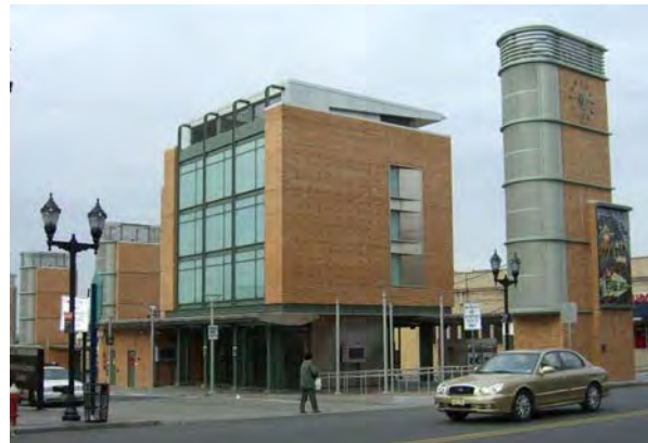
Bergenline Avenue Station
