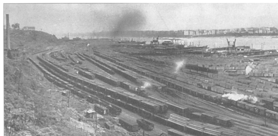
West Shore Freight terminals and grain elevators (New York Central Lines). Considerable freight for the Allies was shipped from these yards.
